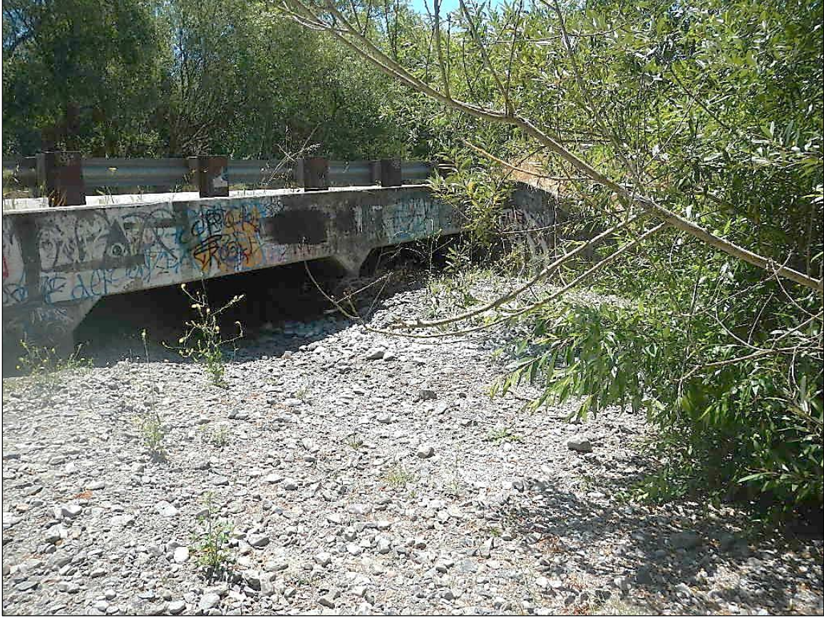
Figure 2.10. Adobe Creek crossing on Casa Grande Road where sediment consistently collects and creates concern for flood management during large storm events.
