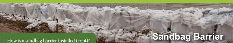
**Selecting Treatment Areas:** Begin by trying to direct debris flows away from buildings and other structures. Clear a path for the debris. Do not try to dam it or stop it. Protect your most valuable property first. Debris can enter a building through doors and windows. They should be boarded up and waterproofed with plastic sheets. Sandbags will not seal out water.
