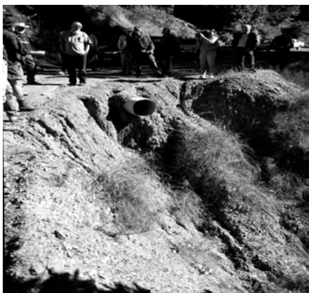
Photo: Typical Erosive impact from rural roads. The culvert is set too high in the bank fill and is undersized for the flow it handles.
